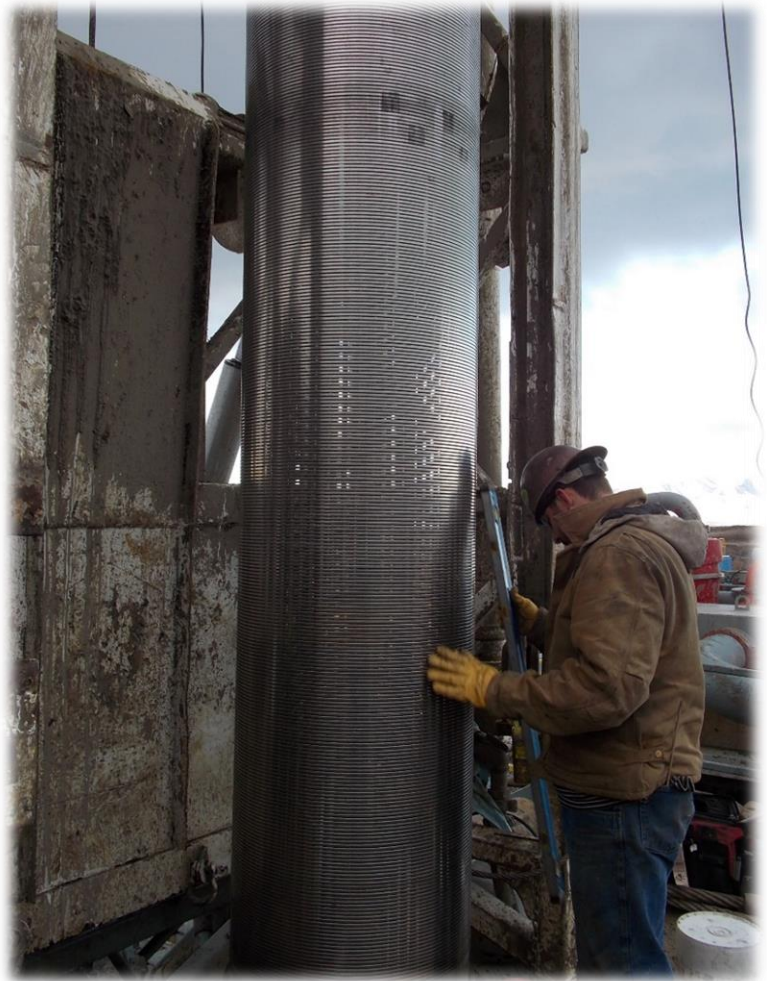
Completion of 600 m deep well using 24-in Super Vee screen
