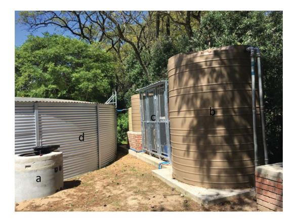
Figure 1: Groundwater supply system (a) borehole equipped with submersible pump (b) raw water tank (c) water treatment (d) water storage tank.
