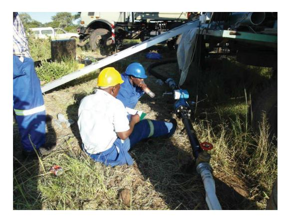
Figure 14: Taking readings from the in-line flow-meter (photo credit: Hans Beekman)
