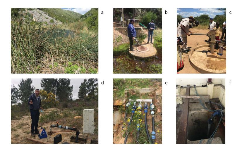
Figure 17: Type of groundwater schemes (a) and (b) spring supplying a town; (c) handpump supplying a village; (d) and (e) cluster of boreholes forming part of a wellfield; and (f) deep well supplying an island community
