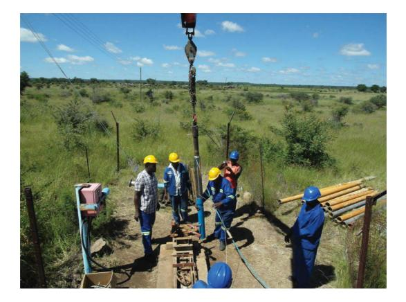
Figure 10: Installing a submersible pump in borehole 64 in the Nyamandhlovu area for pumping tests (photo credit Hans Beekman)
